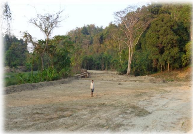
Photo: Tlankima WRC -After Completion
